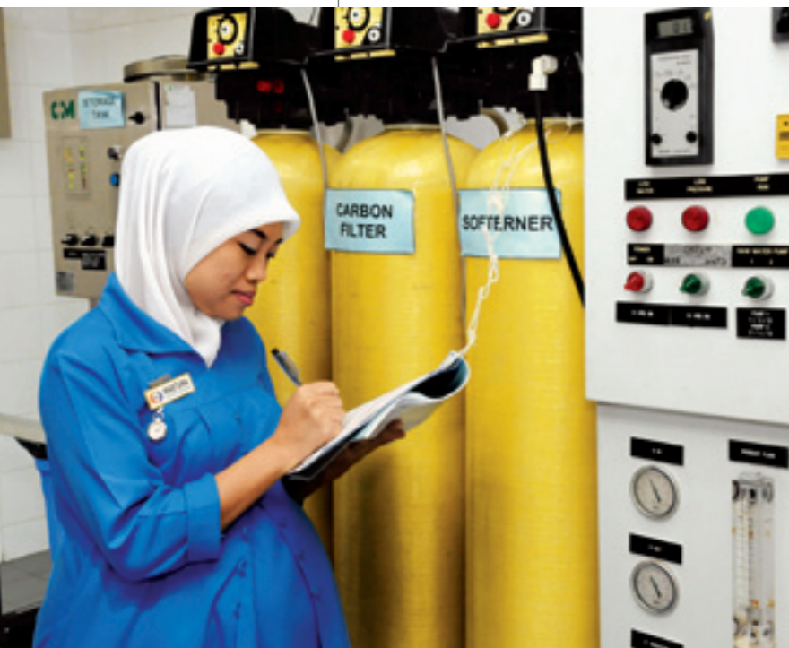
Staff Nurse, Mastura Anwar, performing the regular morning check inside the Reverse Osmosis room. This daily routine ensures proper water purification
